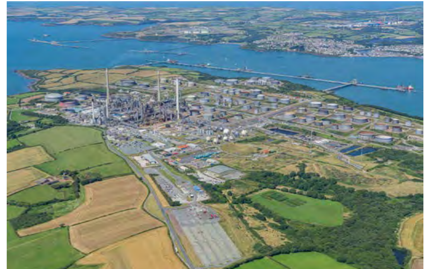
Aerial Views of Pembroke Dock and Oil and Gas terminals at Milford Haven, Wales, UK © Philip / Adobe Stock
