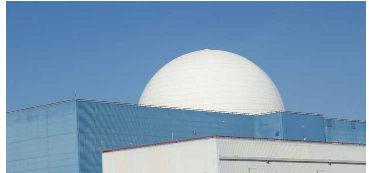
Sizewell B Nuclear Power Station. Photo courtesy of EDF Energy.
