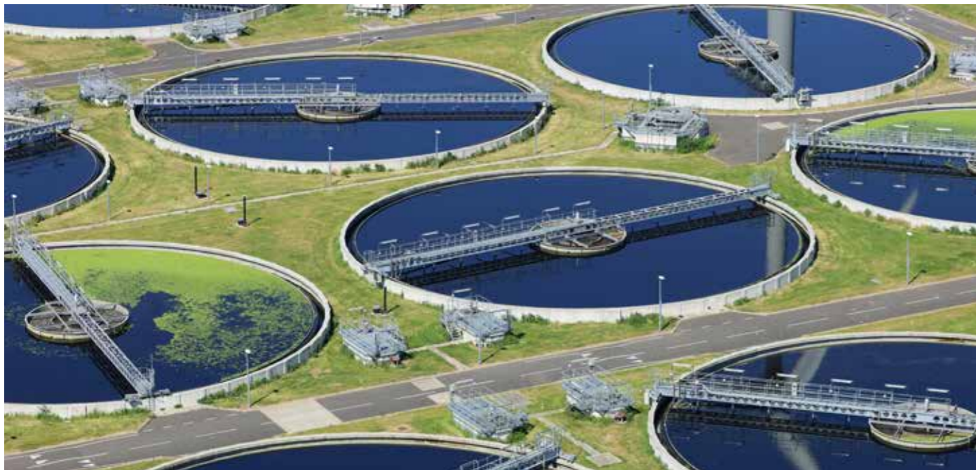
Water treatment facility in East London. © Tom Falcon Harding / Adobe Stock.
